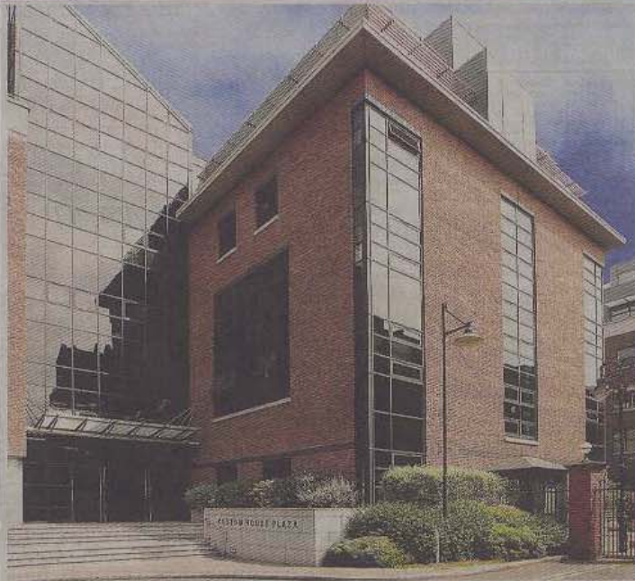
THERE is room at the top — literally — at the IFSC where a stunning penthouse office suite has become available to let at a rent of €505 per sqm per annum. The 269sqm suite is on the fifth floor penthouse of 4 Custom House Plaza. The accommodation includes two boardrooms, a communications room and a filing/storage room. Agent is Jones Lang LaSalle. The space is available immediately on flexible lease terms and comes with car parking at €3,750 per space per annum. JLLS is also marketing a fully fitted second floor office (1,325sqm) in East Point Business Campus at the edge of Dublin's central business district at a rent of €747.50 per sqm per annum.
