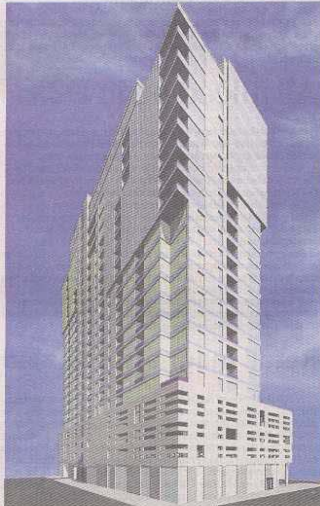
Sean Conlon is developing 640 West Washington in downtown Chicago. The high-rise tower will provide more than 24,100 sqm of accommodation, including both commercial space and 220 units. Walgreens is the anchor tenant
